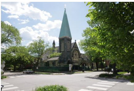
Greenstone Methodist Church
